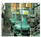
labour and electricity [and] the blockages and leaking glands with the original pumps have been eliminated."
